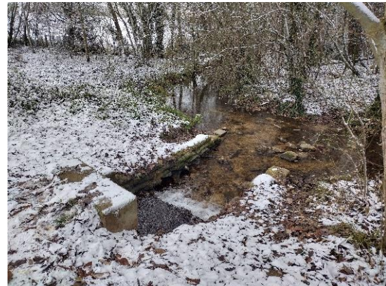
Figure 2.19 Outfall from Trow Pool (looking downstream at SP 54647 24893)
