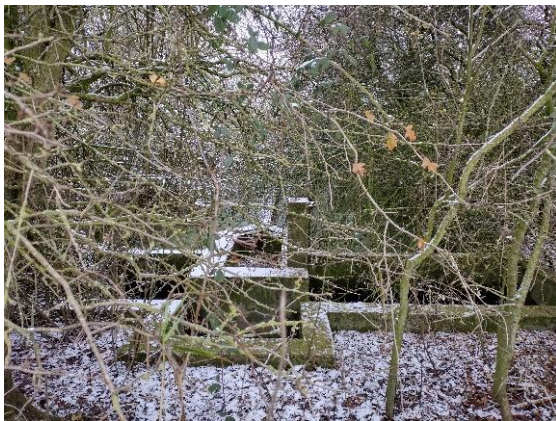
Figure 2.6 Channel source – impounding dam and sluice structure (looking upstream at SP 53289 26850)
