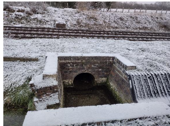
Figure 2.25 Culvert under railway (looking downstream at SP 53131 27573)
