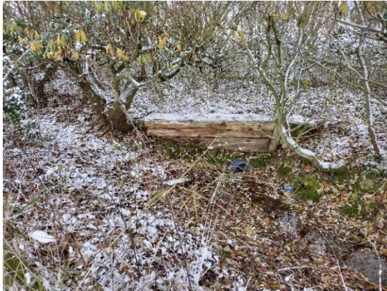
Figure 2.3 Inlet pipe (looking downstream at SP 52927 26132)
